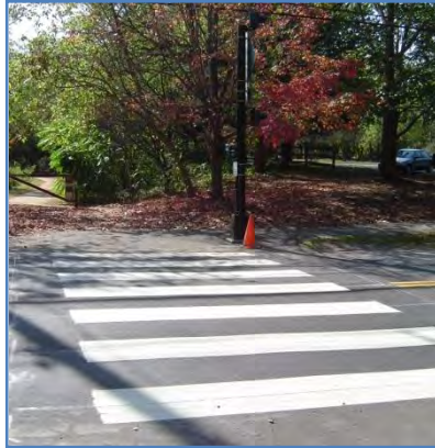
High visibility crosswalk at roadway crossing for the D&R Canal towpath
