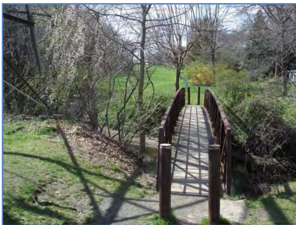
Pedestrian bridge stream crossing
