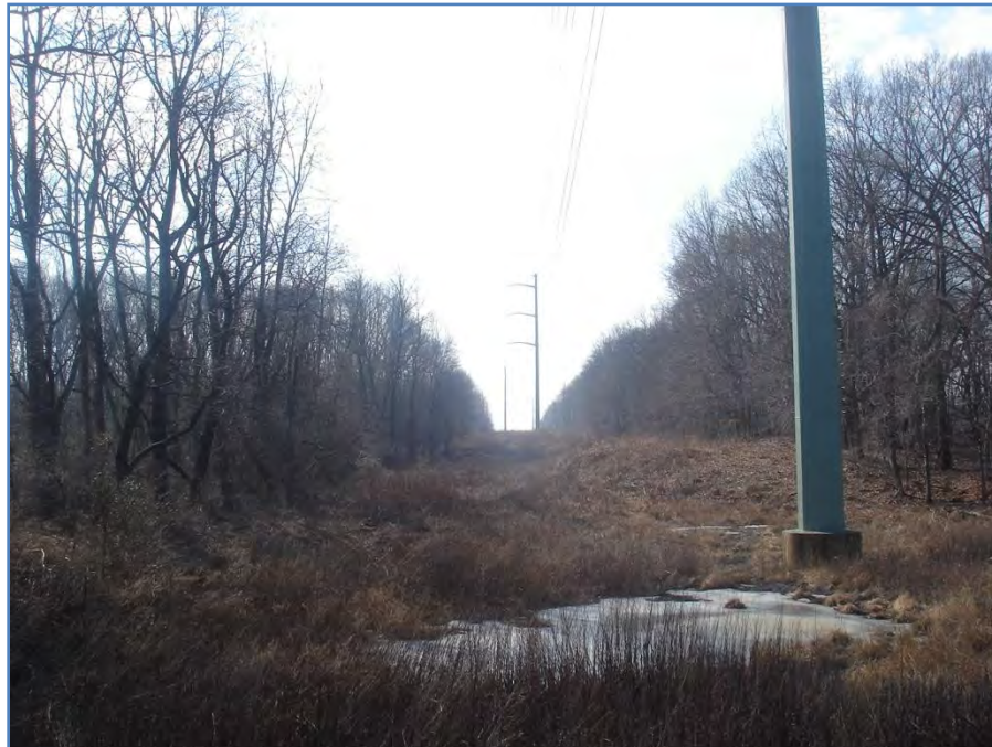
Section of a utility corridor included as part of proposed PSE&G ROW trail, near Route 612
