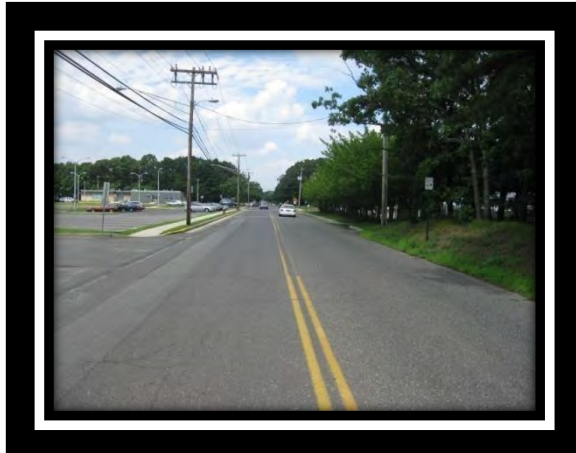
Existing sidewalk on the western side of Monmouth Road south of the Community Center
