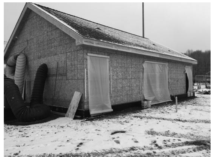
Photos of Daniel Ryan Field's concession and restroom construction.
